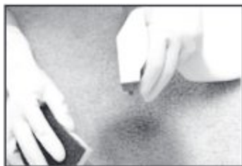
Removing iron stain
