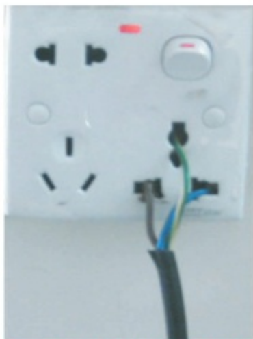
Dangerous/risky electric connection Proper and safe electric connection
