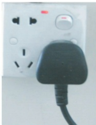
Dangerous/risky electric connection Proper and safe electric connection
